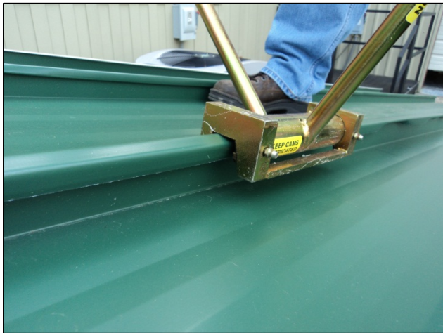
Figure 12-10 Hand-Seamer/Crimper
