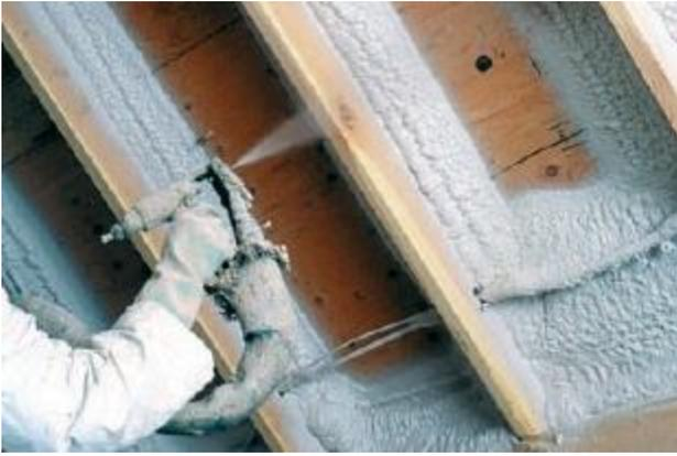
Photo of SPF being applied to wood deck using picture framing technique. Spraying foam onto a metal panel surface would be done in the same fashion.
