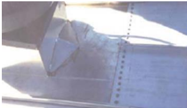
Figure 6: This curb has 12” of clearance between the panel ends and the water diverter, which prevents water buildup.
