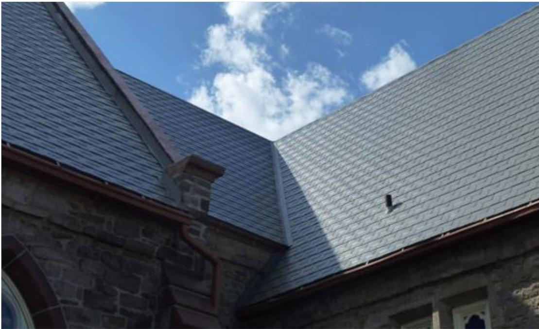
“The ADVANTA shingles have some of the longest life expectations of any roofing product out there,” Bush said. Not only is the product more durable than slate shingles, it is also lightweight, which minimizes the stress on the overall structure.
