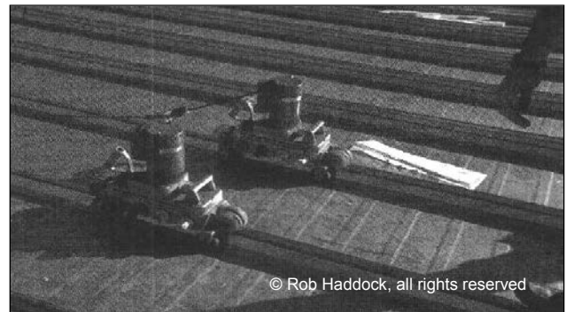
Figure 7-20 Electric Powered Mechanical Seamers Note: Horizontal Ribs on Vertical Panels
