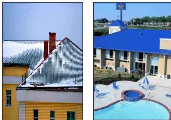
Figure 7-7 Temperature Extremes Are Normal for Any Roof
