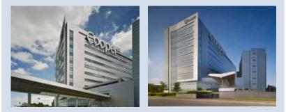
Photos courtesy of EwingCole /CENTRIA IMPs seamlessly integrate with curtain wall and punched windows to provide thermal efficiency and moisture control in a single panelized component.
