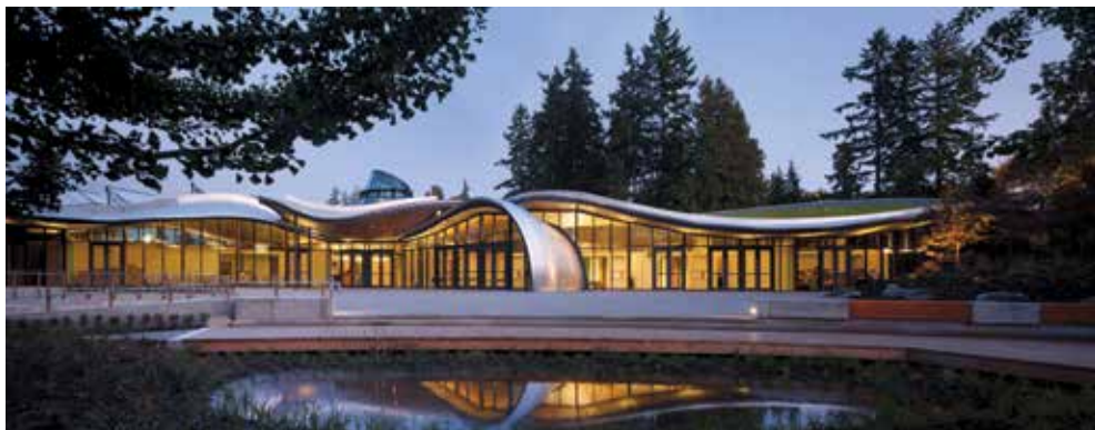
Meeting International Future Living Institute Living Building Challenge standards, the net-zero VanDusen Botanical Gardens Visitor Centre in Vancouver, British Columbia, features a living roof blending striking aluminum composite panels with traditional wood.
