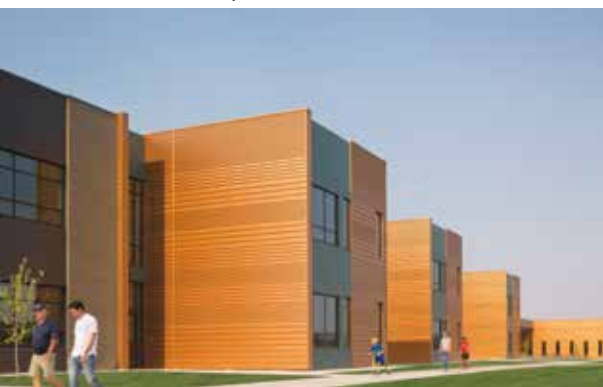
When designing the Medicine Crow Middle School in Billings, Montana, the community was interested in a resilient space that could provide a minimum lifespan of at least 50 years. Sustainable metal wall panels were designed as a durable and aesthetically interesting solution while meeting sustainability and energy goals for the exterior envelope.
