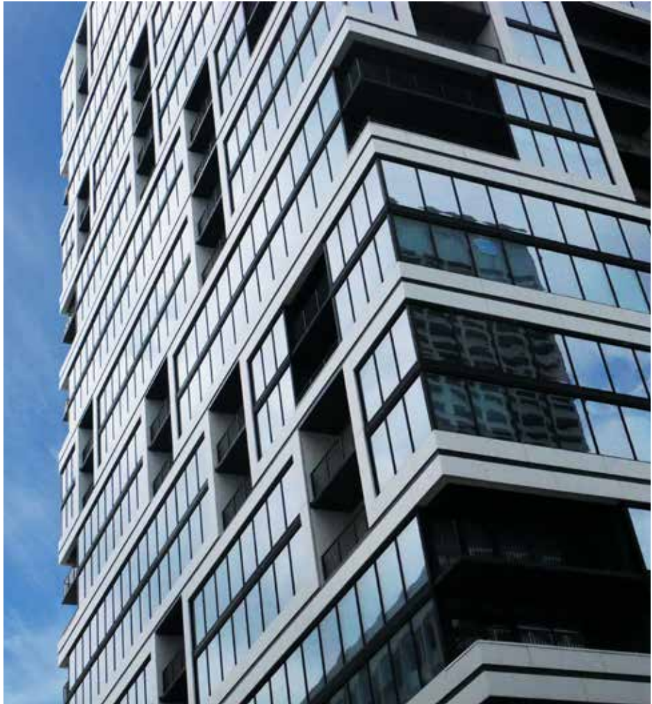
Metal composite material helps create the l's and i's of the lilli Midtown high-end apartment tower in Atlanta.
