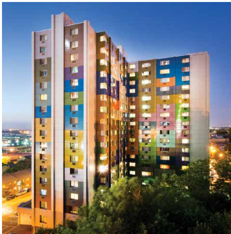
At the Paul F. Cullum Tower in North Bergen, N.J., metal composite material cladding offers a flame-retardant, colorful facade.
