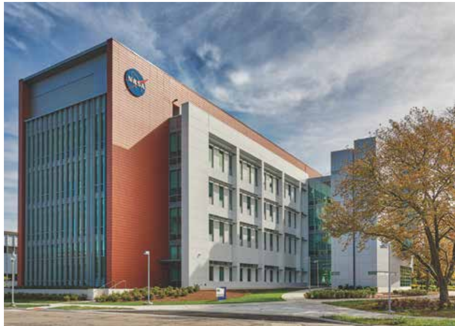
At the NASA Langley Laboratory in Hampton, Va., aluminum composite material in two distinct finishes serve as flame-retardant rainscreen cladding and helps create a modern look for the aeronautic building.
