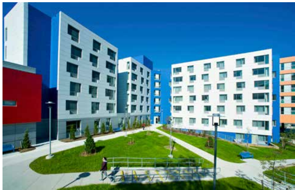
Prefabricated aluminum composite material in bold colors deliver a striking facade at Stony Brook University's Nobel Halls in Stony Brook, N.Y.
