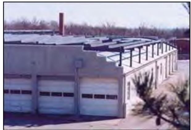
Photo 4-1: Showing how retrofit framing systems can accommodate various existing and problematic roof geometry even with this double-barrel roof. (Courtesy of MBMA)
