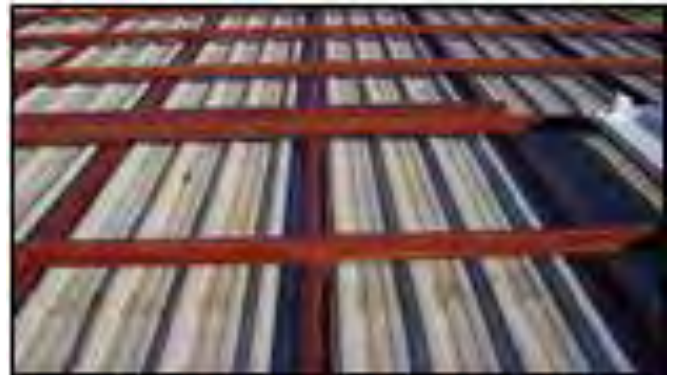
Hat-over-Hat MOM system (Courtesy of Roof Hugger, LLC)
