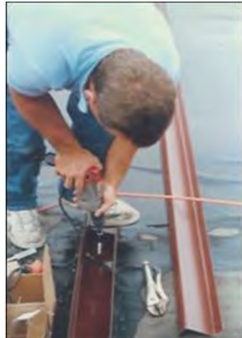
Photo 3-2: Base Channel being installed (Courtesy of McElroy Metal)
