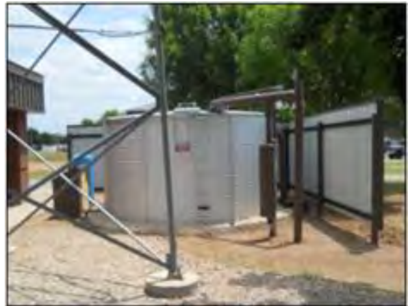
Photo 8-8 – Rainwater above ground storage tank (Courtesy of Roof Hugger, LLC)
