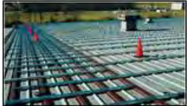
Zee-over-Zee MOM system (Courtesy of MBCI)
