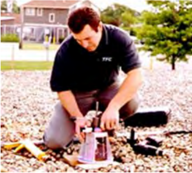
Photo 5-2: Pullout Test being performed on existing BUR flat roof – Photo courtesy of Triangle Fastener Corp.
