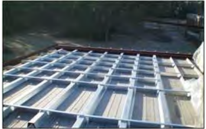
Reinforced corner zone framing (Photo courtesy of Roof Hugger, LLC)
