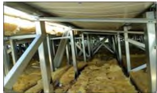
Photo 8-2: Unfaced Fiberglass Installed Over Existing Roof (Courtesy of MBCI)
