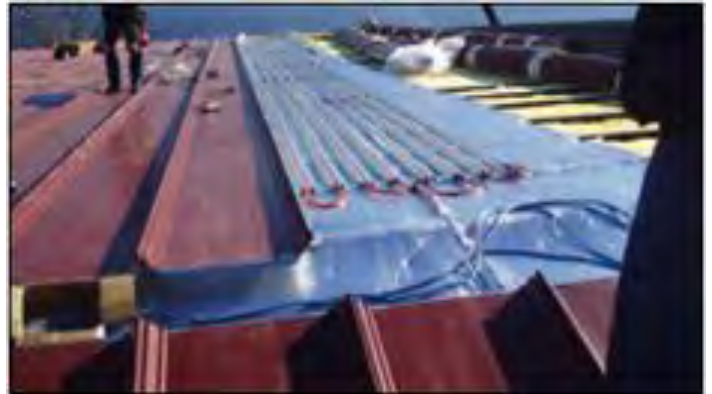
Photo 8-7: Closed Loop Solar Thermal Hot Water System (Courtesy of Roof Hugger, LLC)
