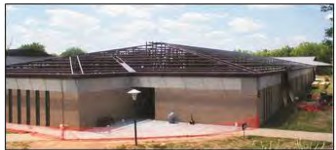
Photo 1-2 Metal-over-Flat Roof System (Courtesy of McElroy Metals)
