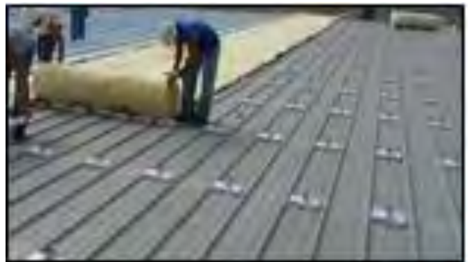
Stand-off clip MOM system (Courtesy of Roof Hugger, LLC)
