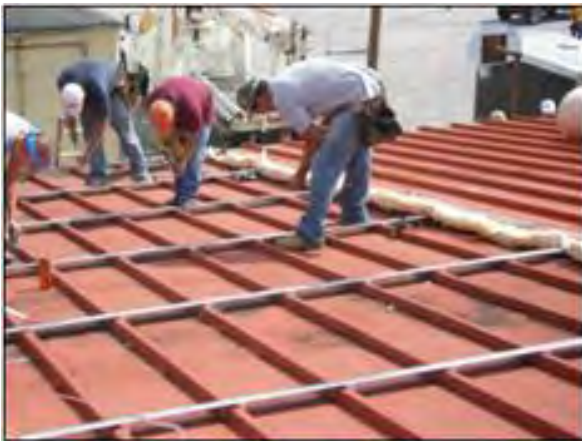
Photo 8-3: Metal-over-Metal Application with Fiberglass insulation (Courtesy of Roof Hugger, LLC)
