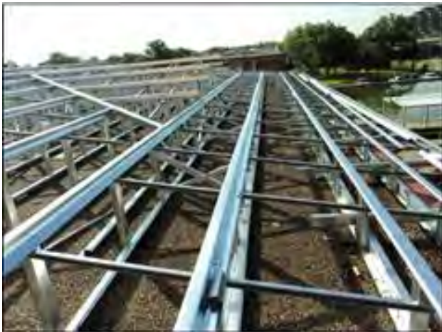
Photo 5-1: Typical Metal-over-Flat roof retrofit system (Courtesy MBCI)
