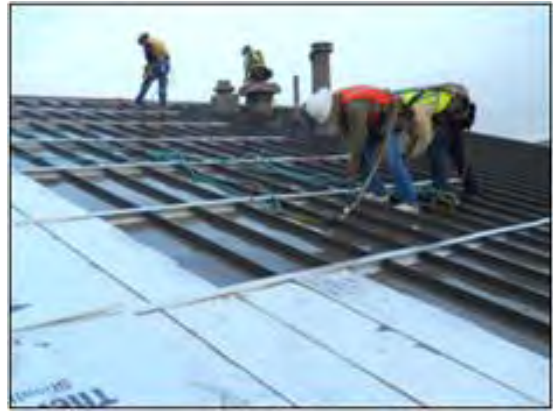
Photo 8-4: Metal-over-Metal Application with Insulation (polyisocyanurate) (Courtesy of Roof Hugger, LLC)
