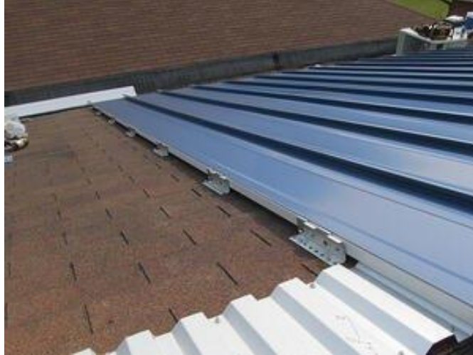
Figure 3: Direct-to-Deck Installation, courtesy of McElroy Metal
