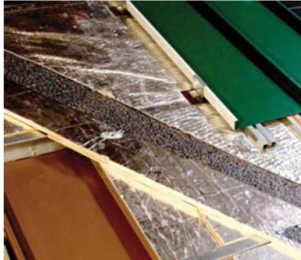
Figure 1: Metal Roof over Radiant Barrier, courtesy of Roof Hugger.
