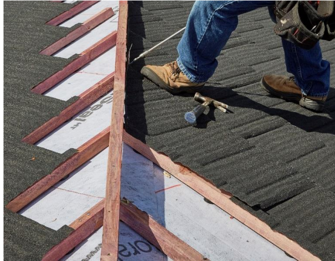
Figure 4: Over-Purlin Installation, courtesy of Boral Roofing
