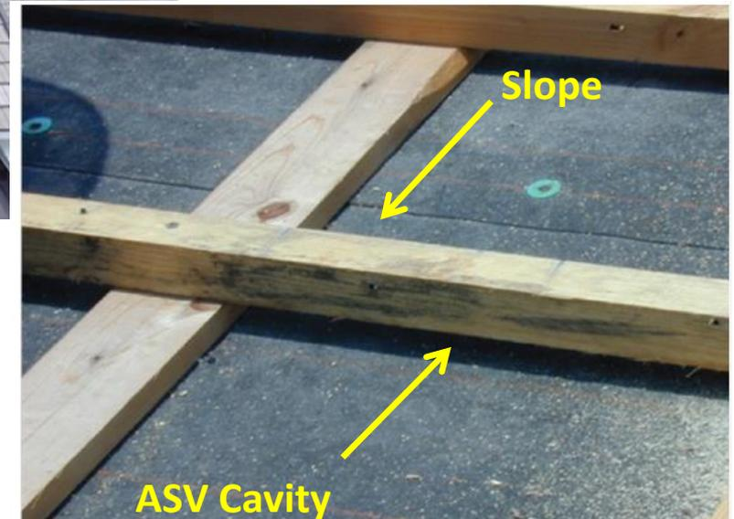
*"A painted metal roof on a 4:12 roof slope with a  $\frac{3}{4}$ " ASV cavity needed only a 0.1 SR to have the same annual cooling load as a 0.25 SR direct-to-deck metal roof"*
