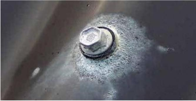
Galvanic Corrosion due to contact of dissimilar metals
