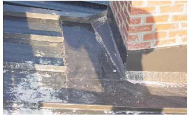
Figure 4. Cement, mortar, and related products can damage metal roofs
