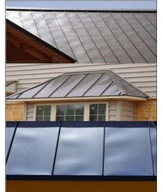
Figure 10-38 Oil Canning of a Metal Roof
