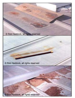
Figure 10-43 Common Debris Can Quickly Damage a Metal Roof
