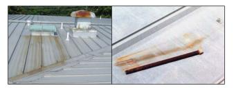
Figure 10-41 Corrosion Damage to a Metal Roof
