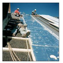
Figure 10-13 Installation of Rigid Polyiso Insulation
