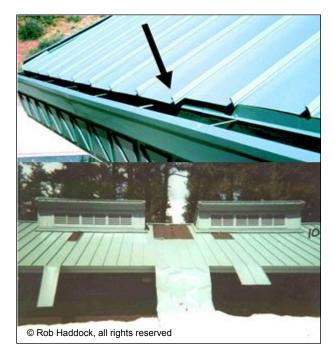
Figure 10-33 Roof Failure Caused by Improper Fixing, or Pinning, of Panels
