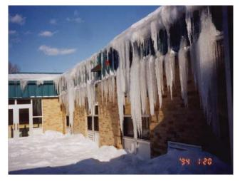
Figure 10-22 Undesirable Ice, Icicles, and Ice Dams
