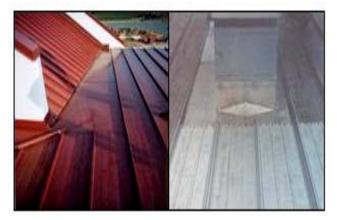
Figure 10-42 Proper Planning and Installation Avoids Ponding Issues
