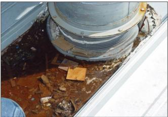
Figure 10-67 Improperly Installed Pipe Blocking Water Flow
