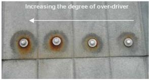
Figure 10-79 Over-Driven Fasteners
