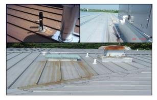
Figure 10-46 Staining and Corrosion from Copper Runoff
