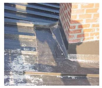
Figure 10-49 Cement, Mortar, and Related Products Can Damage Metal Roofs
