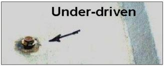
Figure 10-78 Under-Driven Fasteners Will Leak and Corrode
