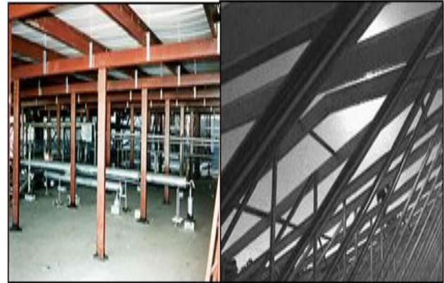
Figure 19-8 Roof Inspections Should Begin Inside the Building
