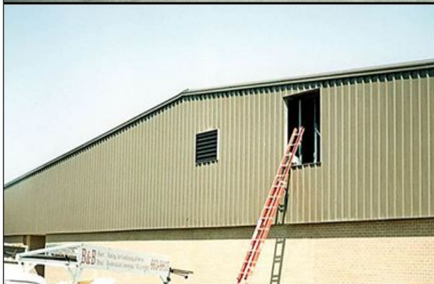
Figure 20-12 Retrofit Endwall Installation
