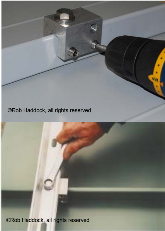
Figure 8-22 Example of Seam Mounted Fence System
