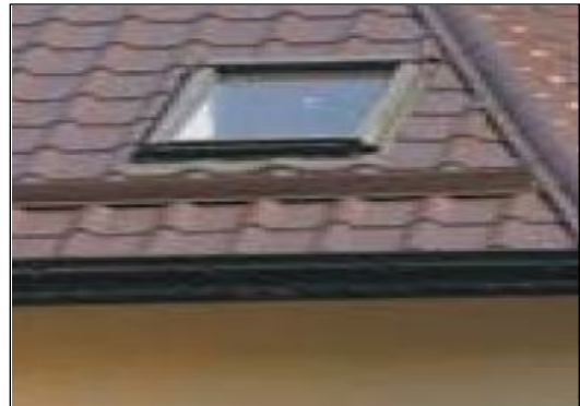
Figure 8-16 Typical Skylight Application
