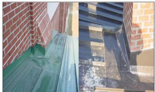
Figure 16-2 Cooperation with Masonry Work Being Performed
