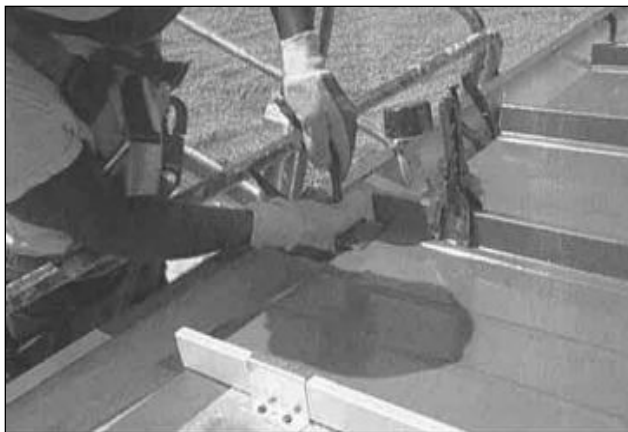
Figure 16-28 Spacer Tools Help Hold Panel Module
