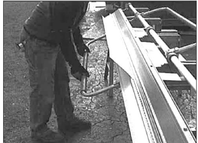
Figure 16-30 On-Site Brake Forming of Roof Material
