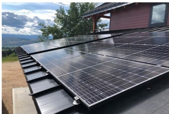
Figure 6: Flush Rail-less Mount (Photo courtesy of S-5!)
