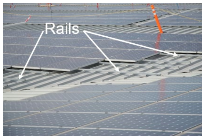
Figure 3: Flush Rail Mounted (Photo courtesy of S-5!)
