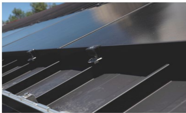
Figure 7: Flush Rail-less Mount (Photo courtesy of S-5!)
