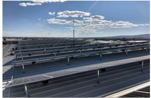
Figure 9: Tilted Mounting System (Photo courtesy of S-5!)
