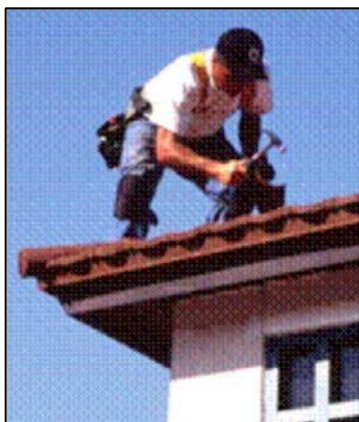
Wide-faced (5-in.) stone-coated or painted metal fascia covers batten framing on roof over applications. The flashing is narrower (3" deep) on new construction.
