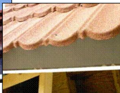
Wide-faced (5-in.) stone-coated or painted metal fascia covers batten framing on roof over applications. The flashing is narrower (3" deep) on new construction.
