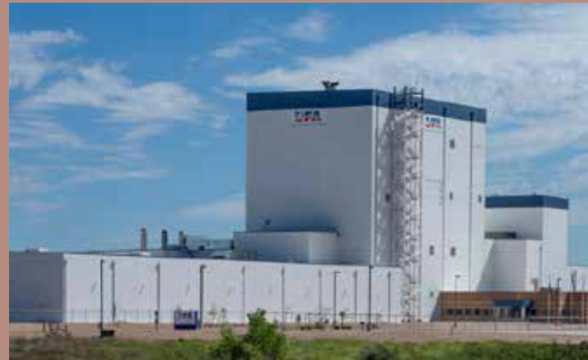
The insulated metal panels on the Dairy Farmers of America facility in Garden City, Kansas, help provide the highest R-value for controlled environment and cold storage needs.
