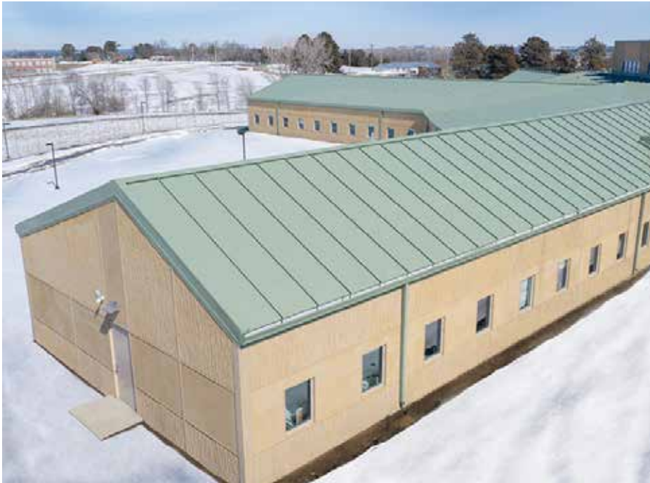
The IMP roofing on Nebraska Correctional Center for Women in Lincoln, Nebraska, provides a low-maintenance, highly energy-efficient solution for the facility.
