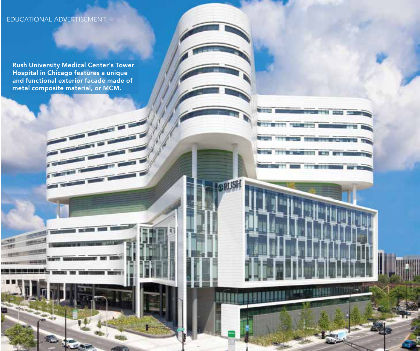
Photo: Robert R. Gigliotti; courtesy of Metal Construction Association
